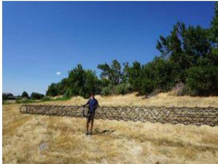
Figure 6. 20-ft IsoTruss sections can be carried and maneuvered by hand rather than needing additional heavy machinery for deployment.
