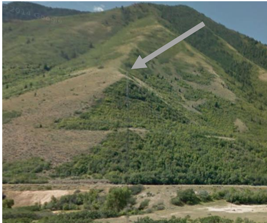
Figure 9. Photograph of an IsoTruss utility pole structure. The lattice geometry of IsoTruss structures causes them to easily blend into the surrounding area. The arrow on the figure points to the IsoTruss structure.
