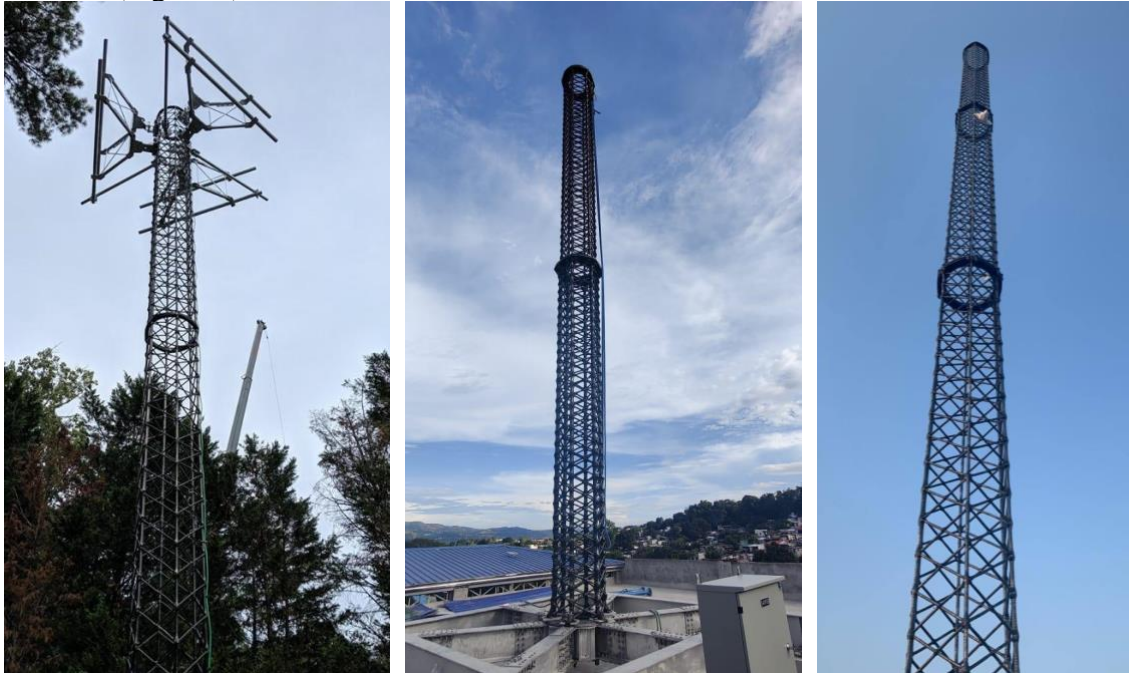
Figure 5. Photos of IsoTruss telecom towers in the USA (left), Philippines (center), and Vietnam (right). All three towers pictured are 40' tall. The tower in the USA was a greenfield deployment and the Philippines and Vietnam deployments were rooftop applications.
